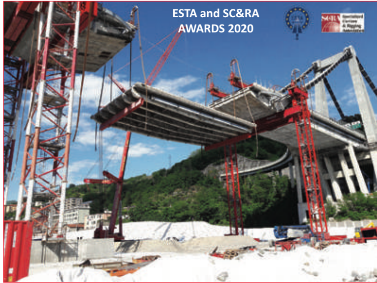
Demolition of Morandi bridge; Installation of the sections of the new S. Giorgio bridge in Genova; SPMTs, Strand Jacks and Crawler Cranes
