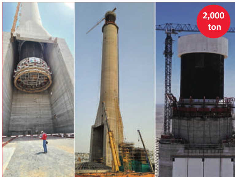
Chile- U.A.E.: Transport, lifting and installation of MSR receivers (2,000 ton) at a height of 200 m by means of skidding and strand jacking systems
